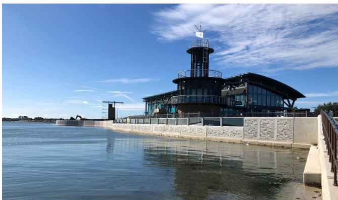
Figure 1. The textured concrete walls will enhance colonisation by marine wildlife.
